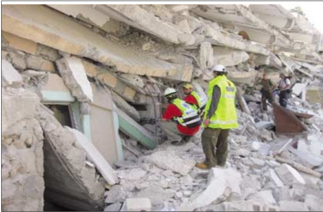
See how the floors just stuck to each other? There are hundreds of bodies in here.
